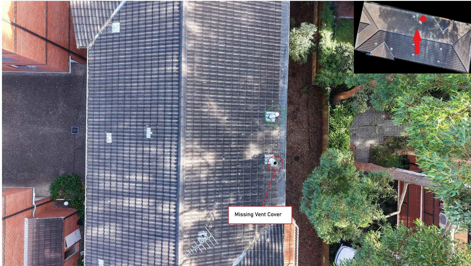
Figure 9 Comments Missing Exhaust Cover
