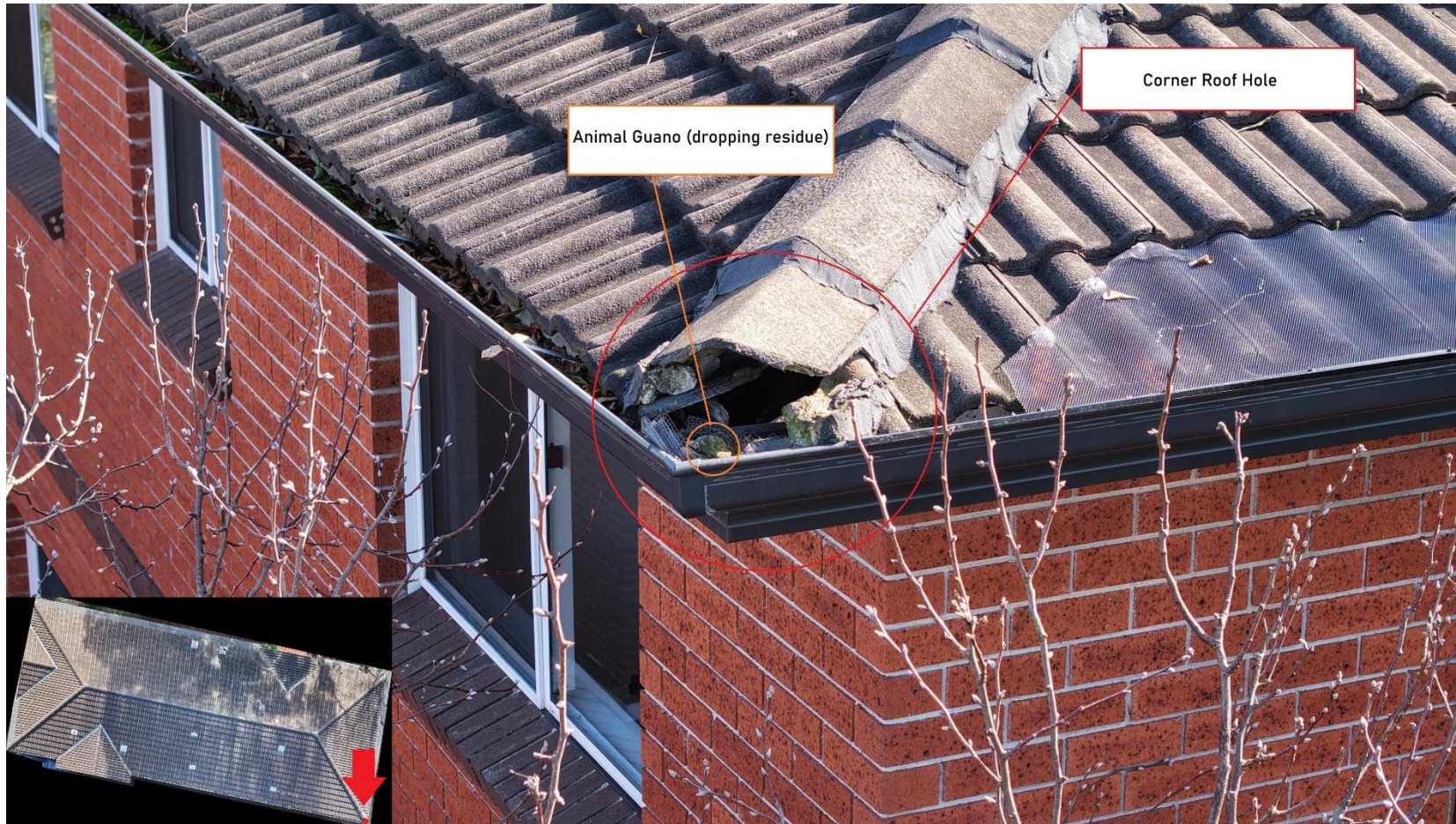
Figure 3 Comments: Clear hole and entry point for wildlife, Tile debris discolouration associated with animal residue
