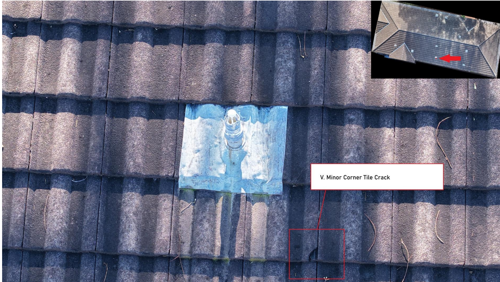
Figure 5 Comments: All Extrusions appeared fine, only this one had a minor crack in the tile
