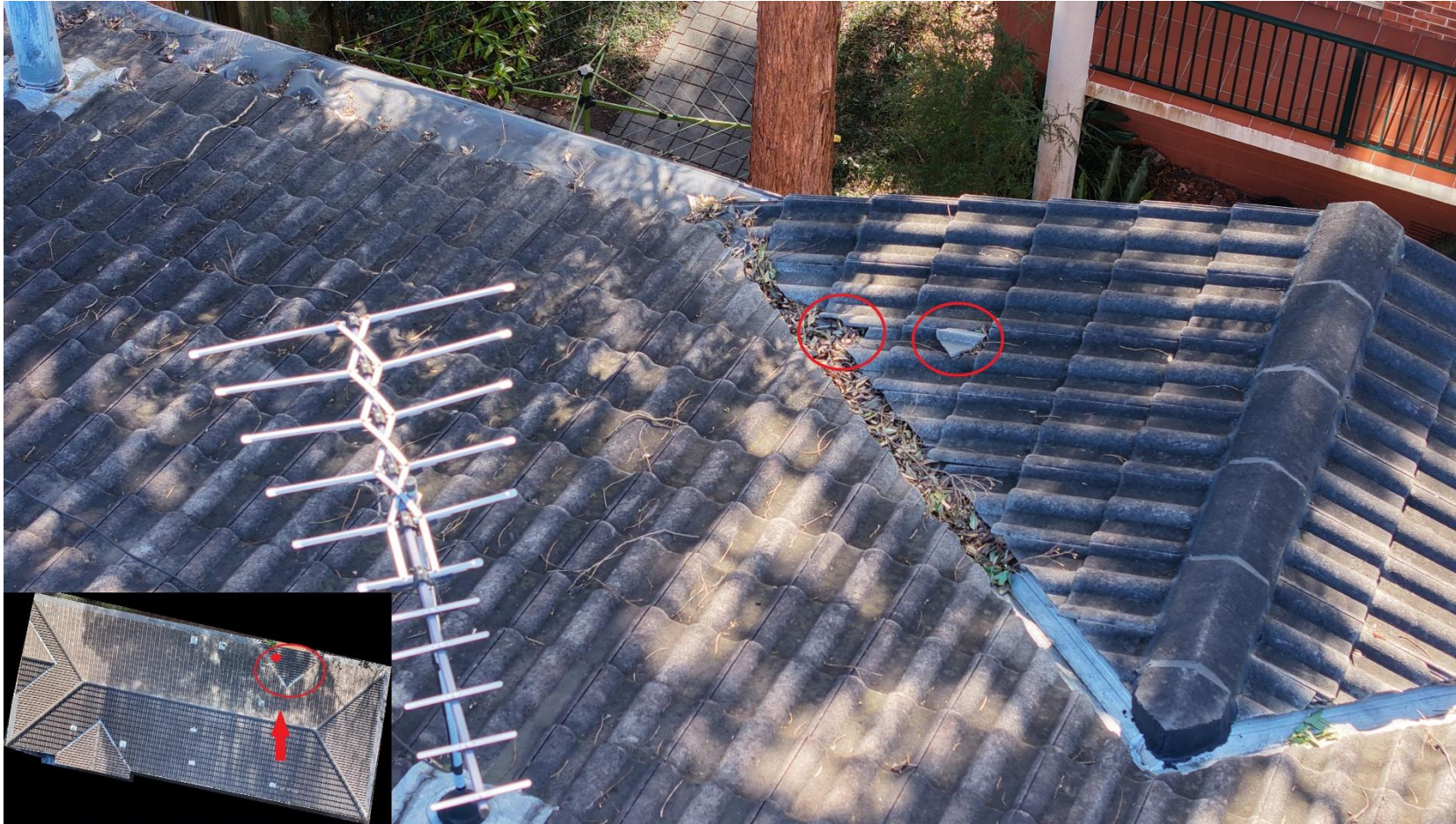
Figure 7 Comments Broken Tile and debris
