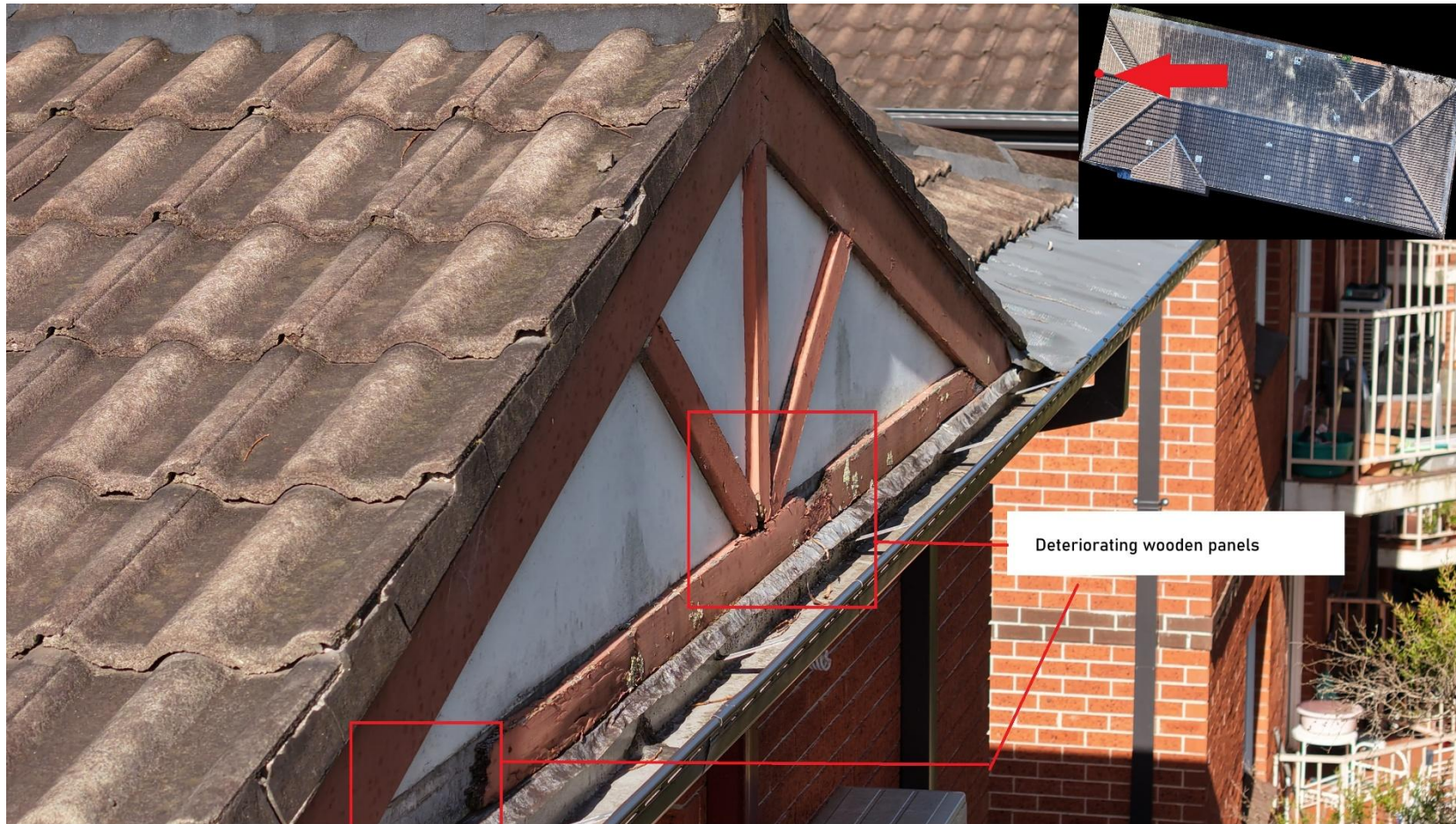
Figure 8 Comments Slight damage affecting the exterior frame
