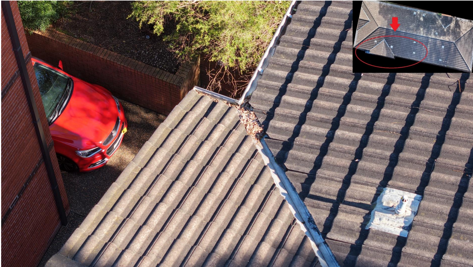
Figure 7 V. small amount of debris, but is present throughout the S and W side of the building
